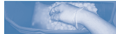
Fig. 7: 'Take away as much as it is necessary to see the bottom of the brine tank'
